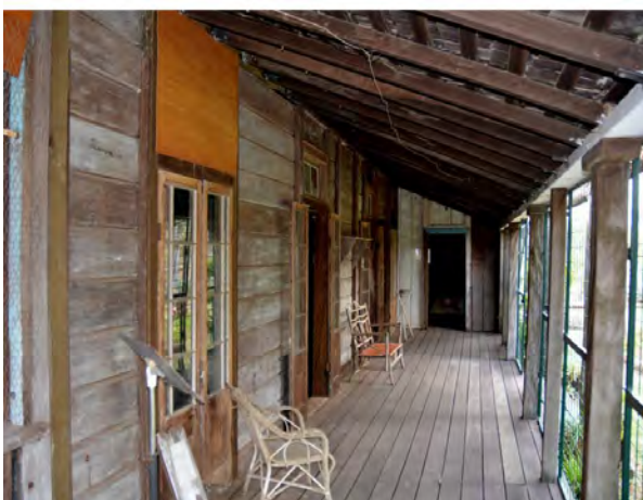
Figure 89. View along the front verandah of the main homestead, showing the French timber doors providing access to the core internal rooms (left) and the bedroom created by the enclosure of the verandah at its western end.
