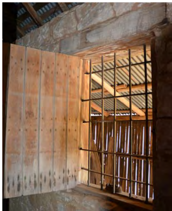
Figure 150. Detail of a typical window shutter made of vertical timber slabs.
