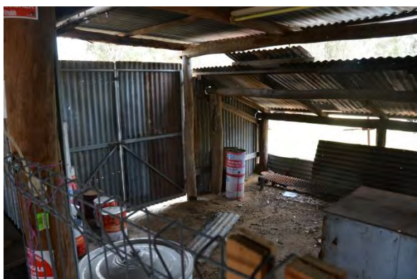
Figure 248. Interior of the rear north-west enclosed skillion extension attached to the camp kitchen.
