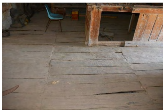
Figure 146. Interior view of hardwood shot-edge boards of the Stone Store.
