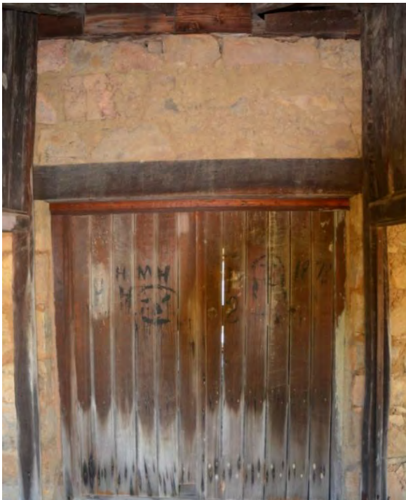
Figure 147. Exterior view of the store's double entrance doors.
