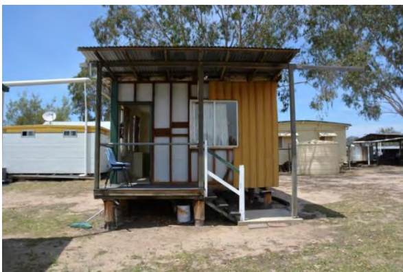
Figure 219. The main north-western elevation of the archives building, showing the external timber stair and landing.
