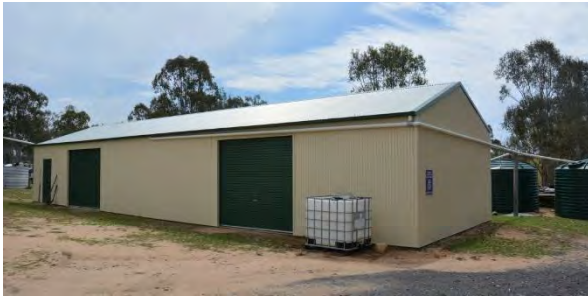
Figure 266. The south-east elevation of the shed.
