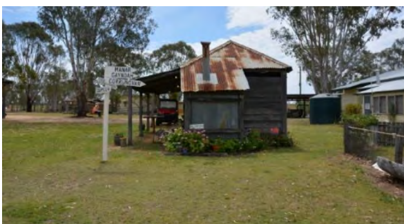
Figure 201. The south-east elevation of Brownie’s hut.
