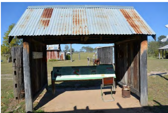
Figure 205. The north-east elevation of the DPI shelter.
