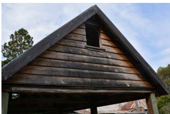
Figure 161. Detail of the timber gable infill.
