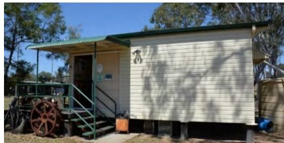
Figure 225. The north-eastern elevation showing the main entrance to the museum building.
