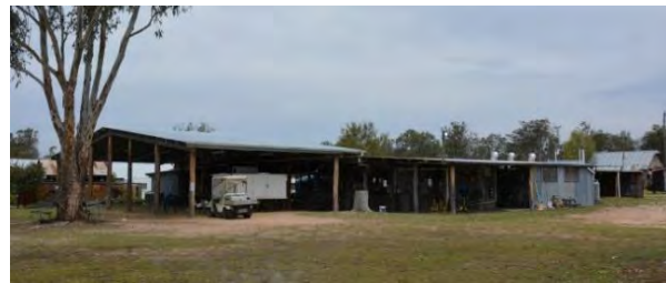
Figure 229. The north-western elevation of the “ entertainment area and extension.
