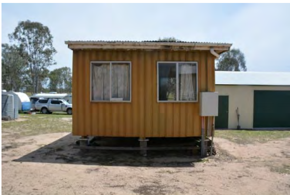
Figure 217. The north-eastern elevation of the archives building.
