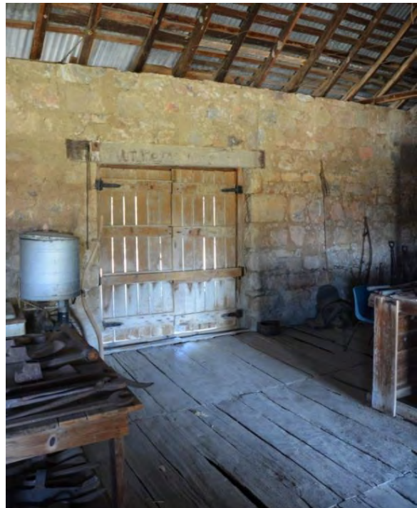
Figure 148. Interior view of the south-west wall of the stone store, showing the floor constructed of wide, hardwood shot-edge boards atop timber joists and bearers, which were restored and reconstructed in the early 2000s.
