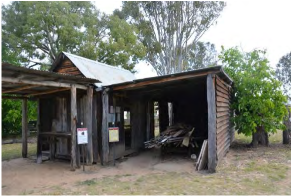
Figure 175. View facing south-west of the postal receiving office showing the adjoining carport extension.
