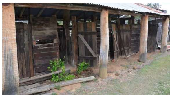
Figure 186. The timber slab doors that divide the milking bails structure internally to create individual stalls.
