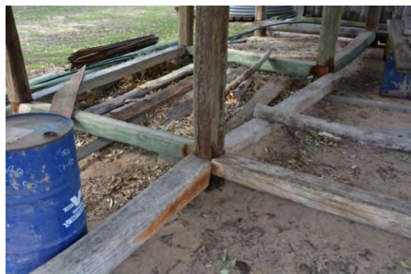
Figure 160. The reconstructed timber bearers and columns comprising the structure.
