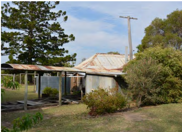
Figure 87. View facing north-east showing covered walkway, constructed of a post-and-sapling frame with a corrugated iron roof, connected to the main homestead.
