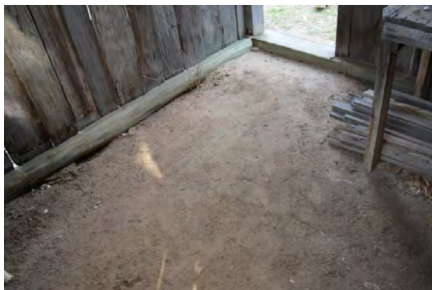
Figure 154. Interior of the meat house showing the compacted earth floor.
