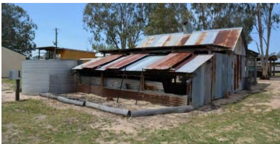
Figure 246. The north-western elevation of the camp kitchen.
