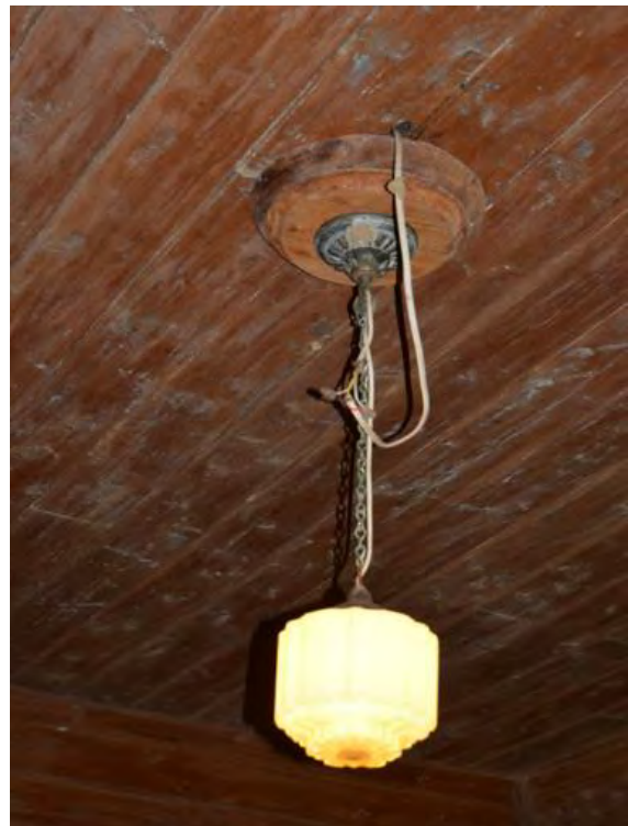
Figure 106. Detail of the single pendant light fitted in the central dining room.
