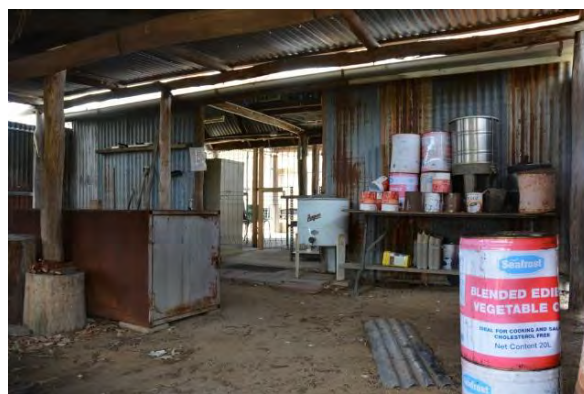
Figure 249. Interior of the main space of the camp kitchen.
