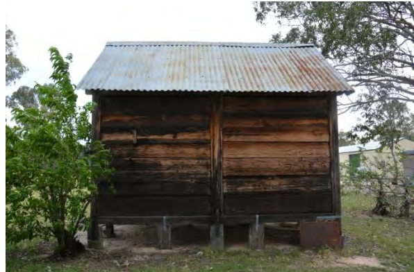
Figure 166. The north-east elevation of the cool house.
