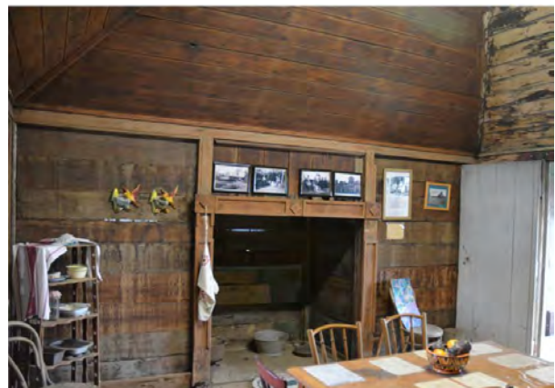
Figure 123. Interior of the detached kitchen, showing the fireplace recess with simple timber mouldings fixed at the joints with the framing.
