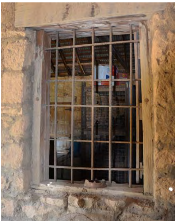
Figure 149. Detail of a typical window with timber lintels and frames and iron bars.
