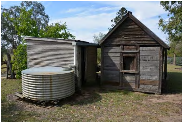
Figure 171. The rear south-west elevation of the postal receiving office, showing the adjacent carport skillion-roof extension and water tank.
