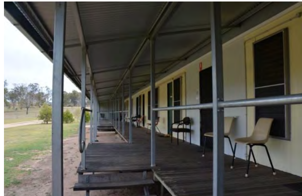
Figure 243. View facing south-west along the front verandah of the accommodation building, providing access to the individual bedrooms, kitchenette and bathroom.
