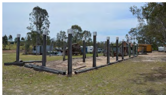
Figure 257. The south-western corner of the former blacksmith's shop.
