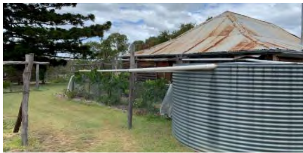
Figure 83. The north-west elevation of the main homestead.
