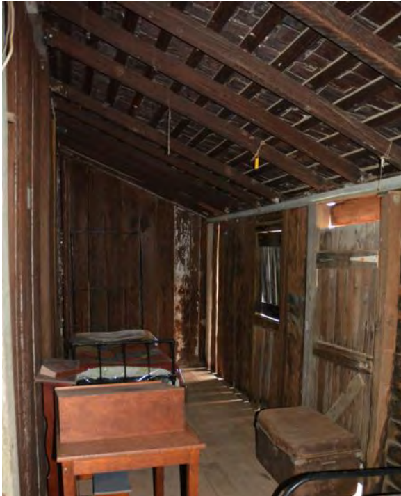
Figure 118. Interior of Bedroom 3, showing the surviving roof shingles fixed under the roof sheet.
