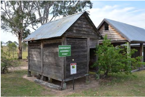
Figure 165. The south-east elevation of the cool house, with the reconstruction of the detached c.1870s 'dining room' structure adjacent.
