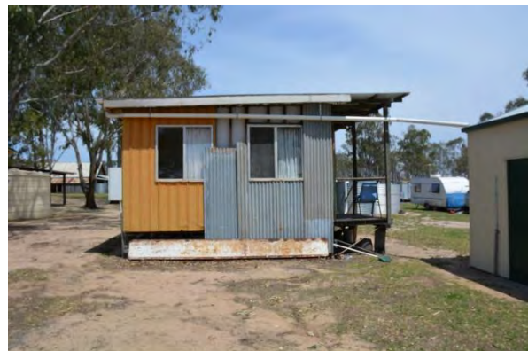
Figure 218. The north-eastern elevation of the archives building.
