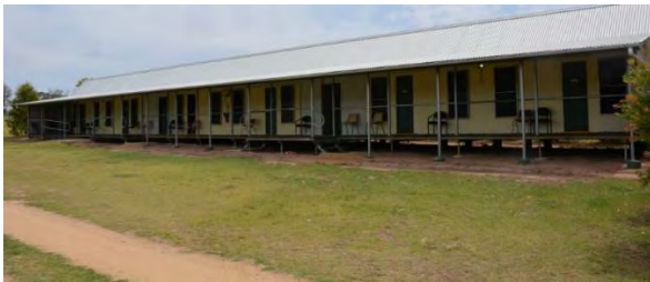
Figure 240. The south-east elevation of the accommodation building.
