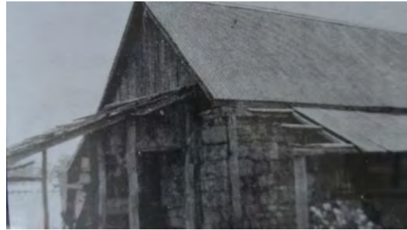
Figure 21. The stone store building c.1949, with the remnants of the timber 'butcher's shop' attached to the south-western façade. Source: Boondooma Museum & Heritage Association (2021).
