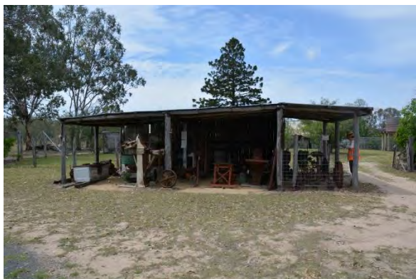
Figure 179. The south-west elevation of the machinery display shelter. Note the timber partitions dividing the shelter into separate sections.
