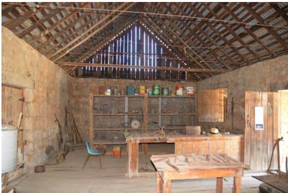
Figure 141. Interior of the north-west end of the stone store. Note the exposed timber rafters and roof framing.
