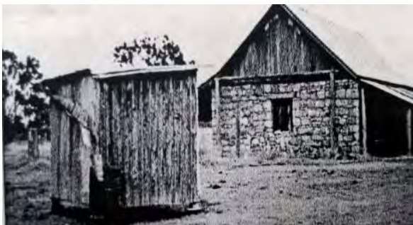
Figure 22. The stone store building (right), with the adjacent boundary rider's hut (left), c.1999. Source: Boondooma Museum & Heritage Association (2021). 27
