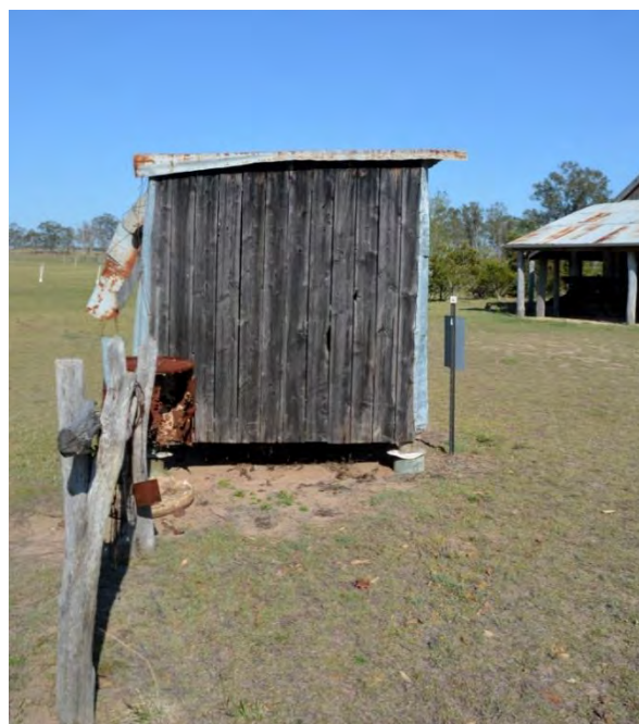
Figure 210. The eastern elevation of the boundary rider's hut, with the stone store building partially visible at the right.
