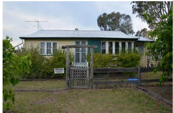
Figure 190. The main north-west elevation of the caretaker's cottage.
