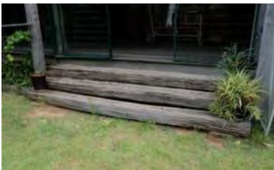
Figure 84. The timber entrance steps providing access to the front verandah of the homestead.
