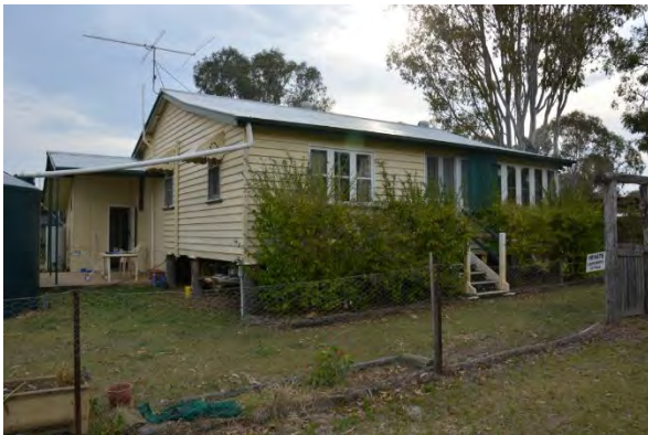
Figure 189. The south-east elevation of the caretaker's cottage.
