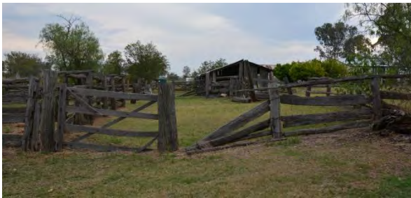
Figure 183. View facing south-west showing the dilapidated section of the stockyards and the milking bails structure behind.
