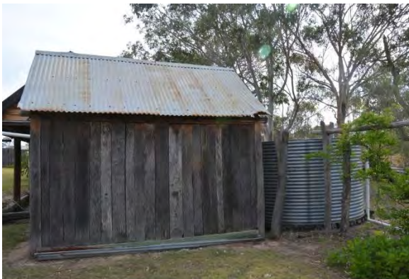
Figure 151. The north-east elevation of the meat house with a large water tank adjacent.
