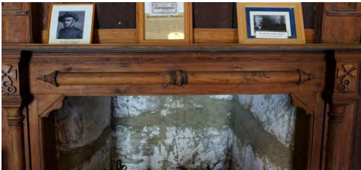
Figure 107. Detail of the timber mantelpiece of the dining room fireplace in the main homestead. Note the finely-detailed timber joinery and mouldings. The early shellack and wax finish of the mantelpiece has been removed.
