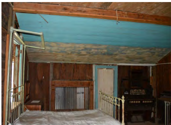
Figure 110. Interior of Bedroom 1 showing the wall under the low side of the ceiling with a small timber slab door that accesses an additional room, which is considered to have been used as a nursery.
