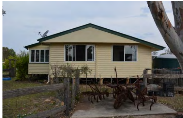
Figure 192. The south-west elevation of the caretaker's cottage.
