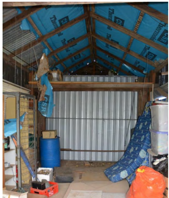
Figure 198. Typical interior of the caretaker's store.
