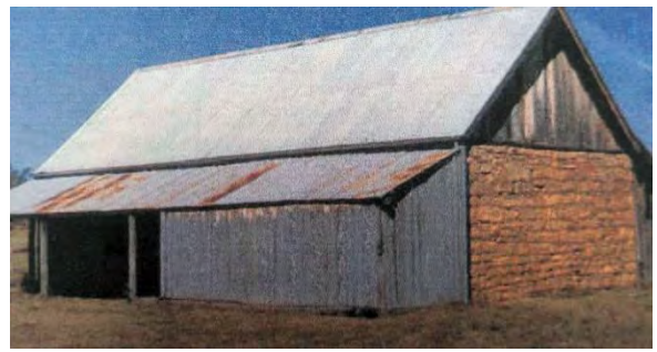
Figure 23. The stone store building at Boondooma, c. 2002. Source: Boondooma Museum & Heritage Association (2021). 28
