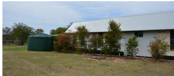
Figure 241. The north-west elevation of the accommodation building.
