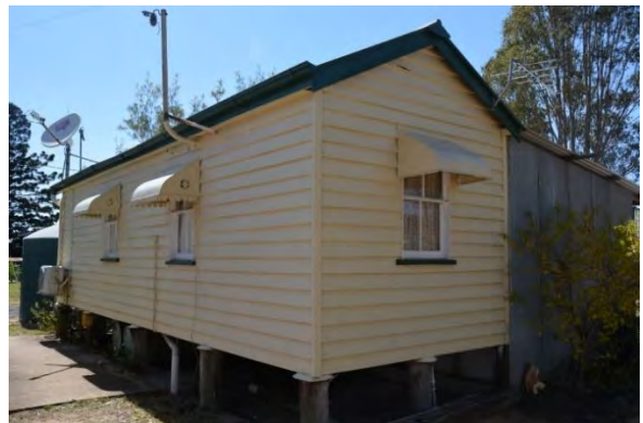
Figure 216. The south-western corner of the administration building.
