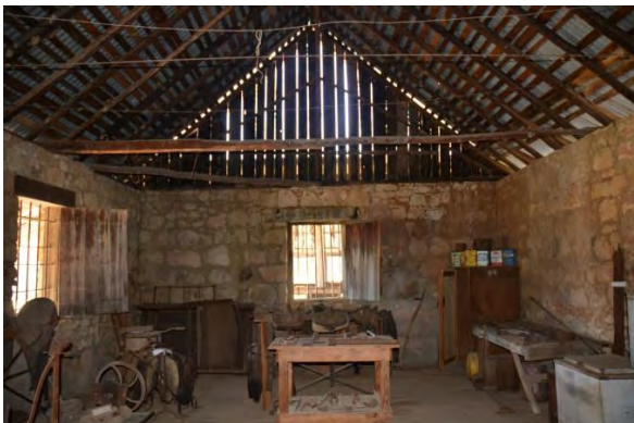
Figure 143. Interior of south-east end of the stone store. Note the two windows with vertical iron bars and timber shutters.
