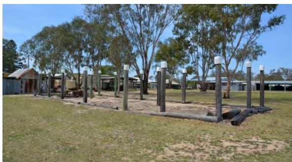
Figure 256. The north-western side of the former blacksmith's shop.
