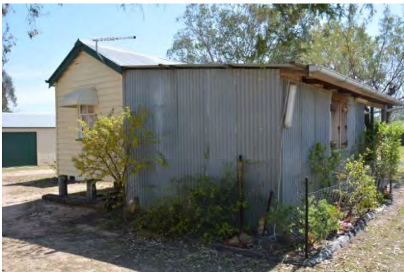
Figure 215. The south-eastern corner of the administration building, showing the corrugated iron skillion extension.
