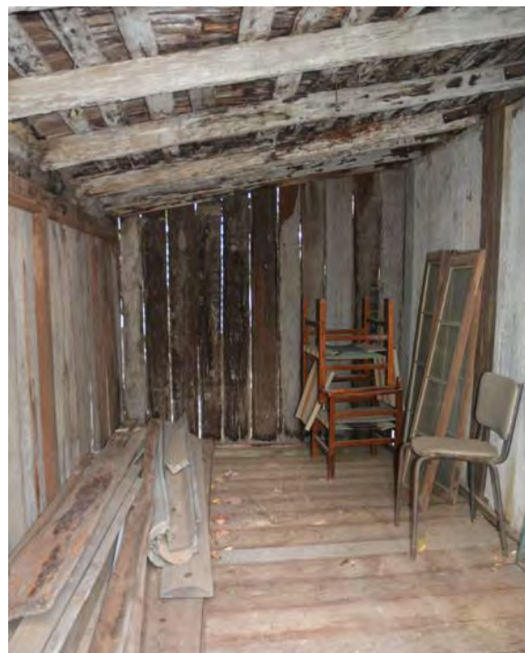
Figure 111. Interior of the addition to the eastern wall of Bedroom 1, which is considered to be a former nursery area.
