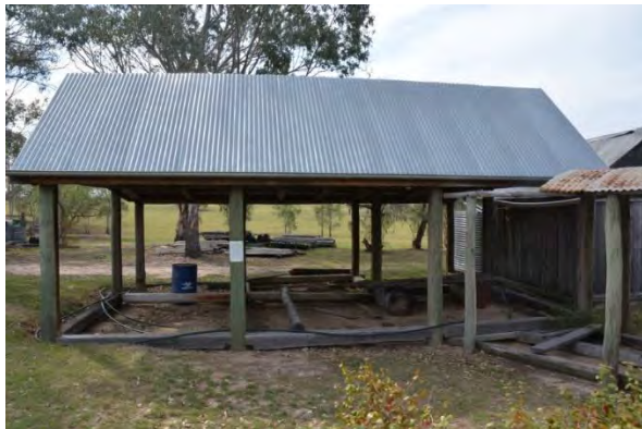
Figure 157. View facing north-west of the incomplete reconstruction of the detached c.1870s 'dining room' structure, or possibly an earlier dwelling.
