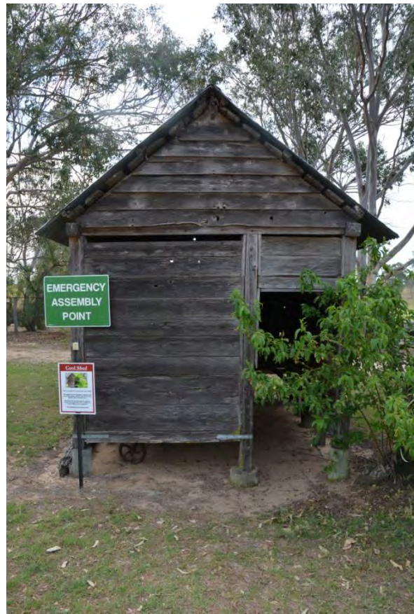
Figure 164. The main south-east elevation of the cool house, constructed of Cypress pine slabs, horizontally fitted.
