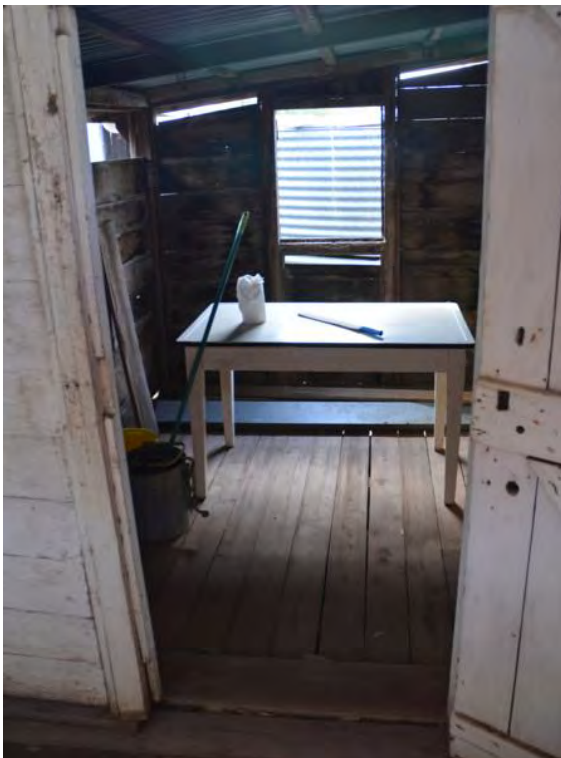
Figure 120. Interior of the small room of unknown use created through the addition of a skillion-roof extension.
