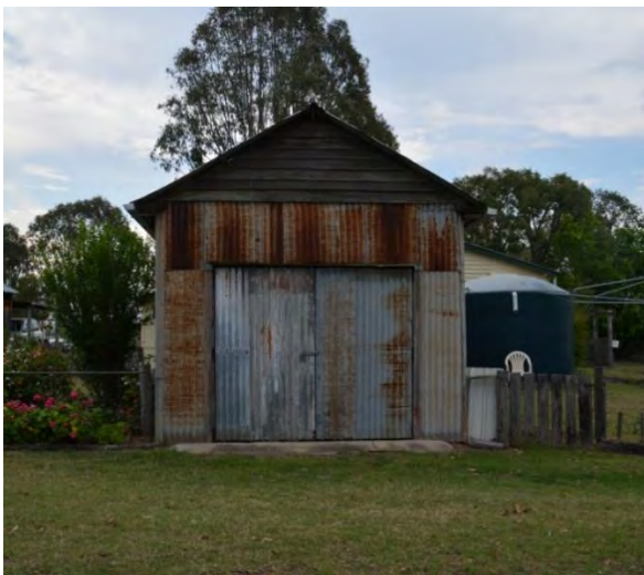
Figure 197. The south-east elevation of the caretaker's store, showing the double door access.
