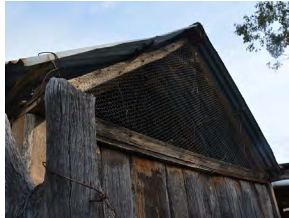
Figure 156. Detail of the chicken wire mesh gable infill.
